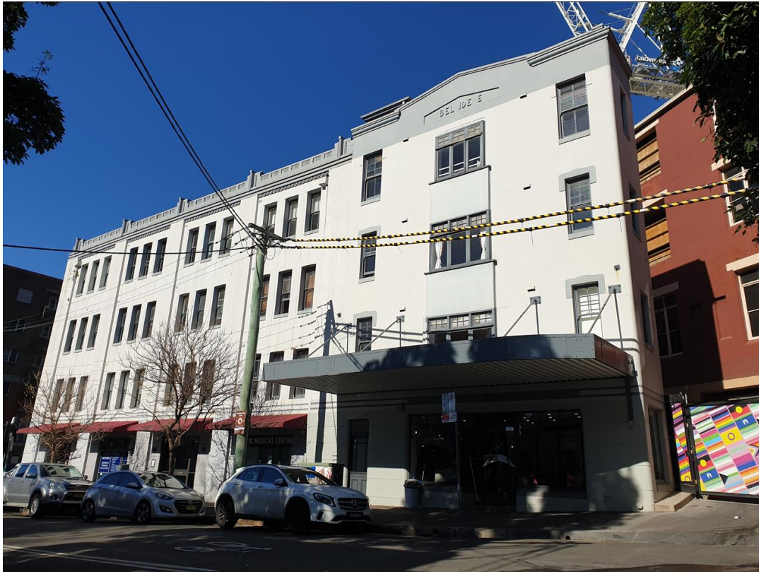
Figure 9: Existing mixed use building at 7-13 Burton Street, Darlinghurst viewed from the northern side of Burton Street adjacent, looking south-east
